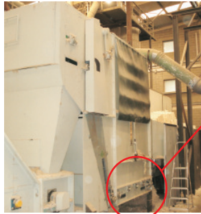
Loader at the back. The apron belt is at the front.
