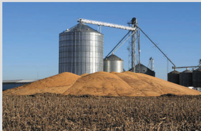
Cereal silos with bucket elevators.
